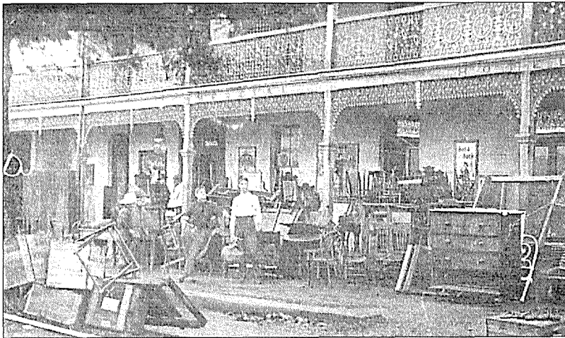
Commercial Hotel after the fire in 1914 or 1915. Many of the furnishings have been removed to the footpath
