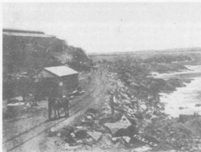
Breakwater construction.
